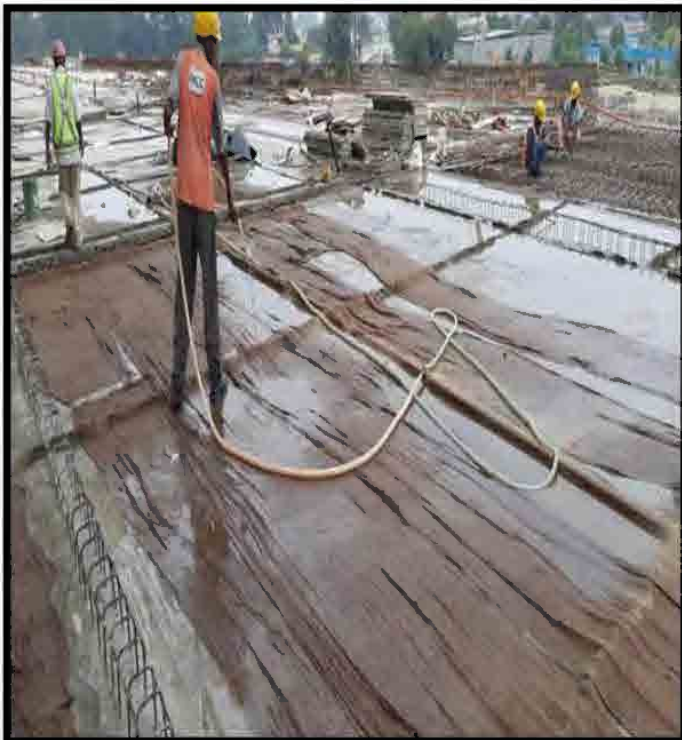
Use of hessian cloth to save water during concrete slab curing
