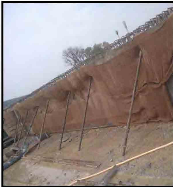
Use of hessian cloth to save water during concrete slab curing
